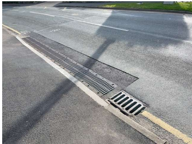
Figure 25 - Additional drainage installed
