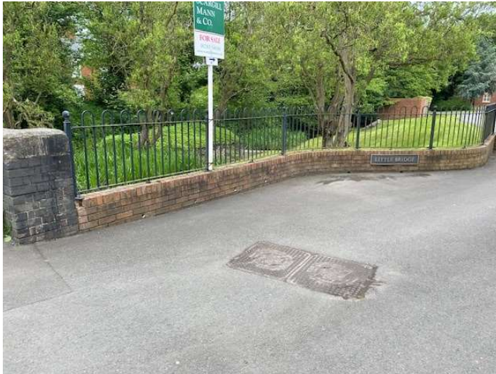
Figure 23 – Feature potentially holds back water
