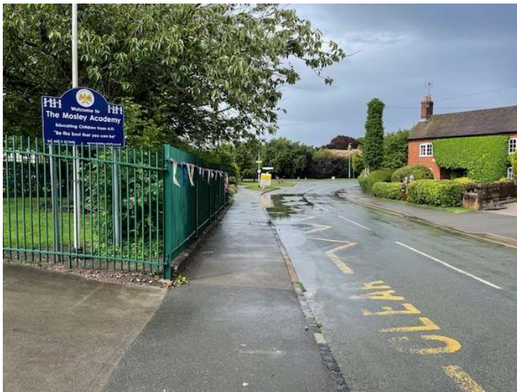
Figure 18 – Flooding from gully outside The Mosley Academy
