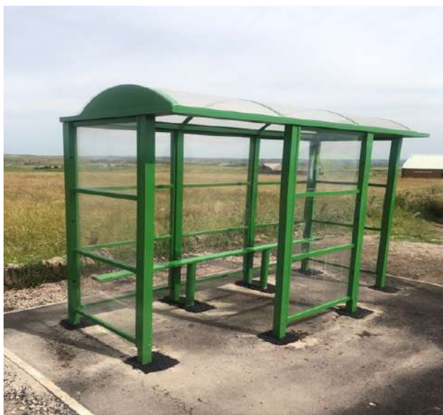
Figure 7: 3-Bay, Enclosed Bus Shelter
