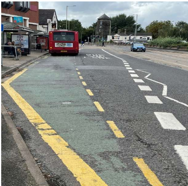
Figure 12: Bus & Cycle Lane - Chell Road, Stafford
