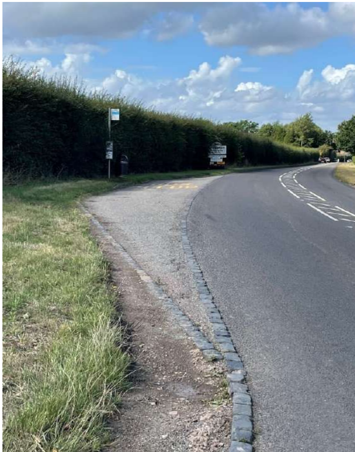
Figure 8: Bus Layby, Westbound - Haughton, Staffordshire
