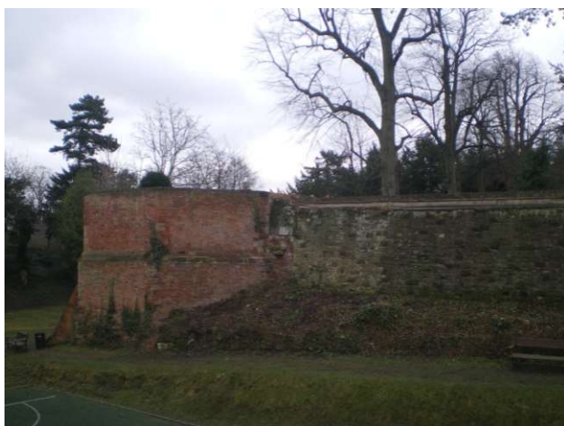
Plate 24: Moat and boundary wall
