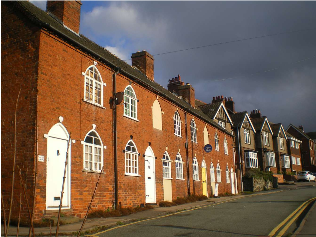
Plate 28: Levetts Fields: Terraces of circa 1830 in foreground and early 20th century properties beyond
